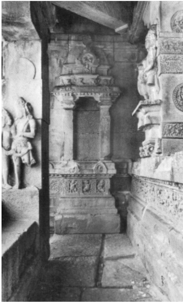
12. Photograph by Gary Tartakov showing cracks in porch floor before the niche to the left of the entrance.
