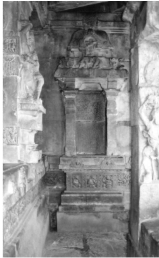
13. Photograph by the author showing mortar filled cracks in the porch floor before the niche to the right of the entrance.
